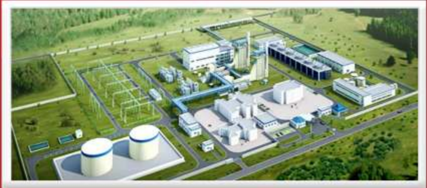
225 MW COMBINED CYCLE POWER PLANT OF SAIF POWER LIMITED LOCATED AT QADARABAD, DISTRICT SAHIWAL, PUNJAB, PAKISTAN
